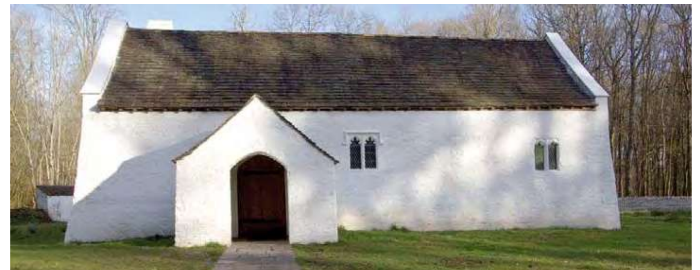
St Teilo's church in which underfloor heating has been installed.
