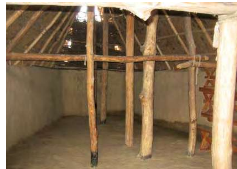
Which roof supports are from the same time period?
