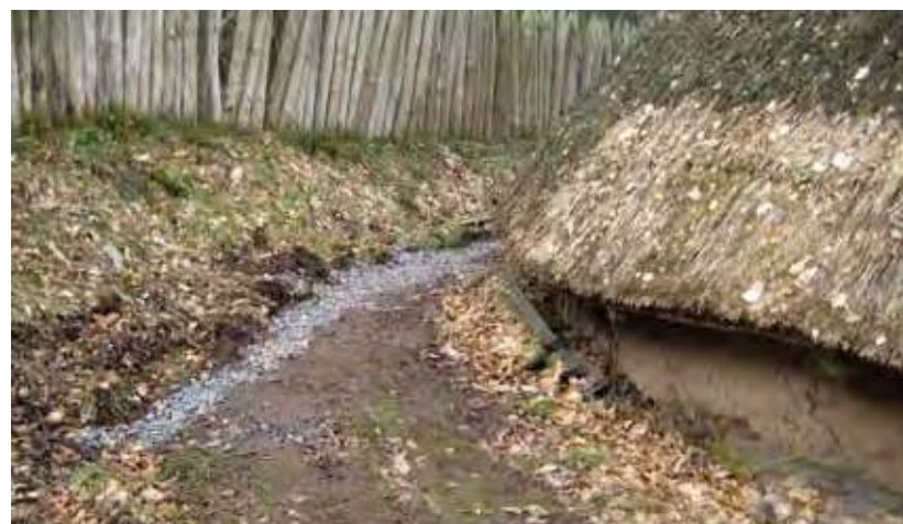
Wet area around the round house ruin the building.
