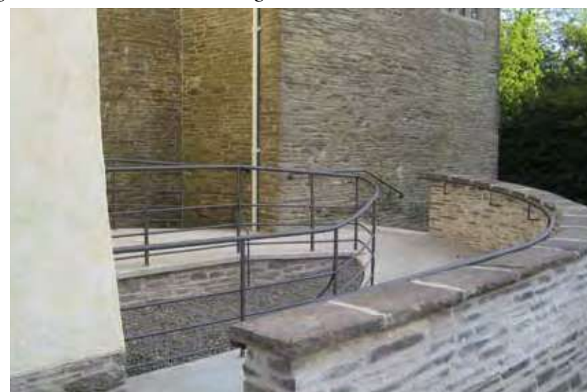
Ramp that blends in with the historic environment.
