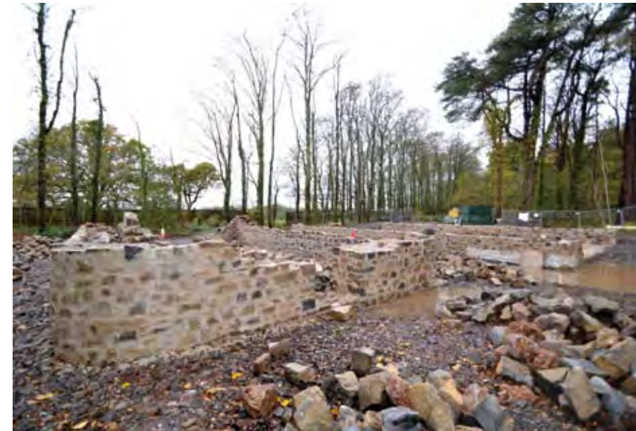
The ground plan of the larger of the two buildings at any early stage in the construction.
