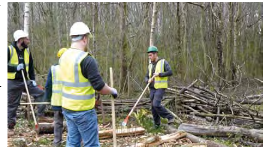
Volunteers removing bark from roof timbers.
