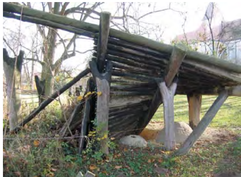
Reconstructed house in decay.
